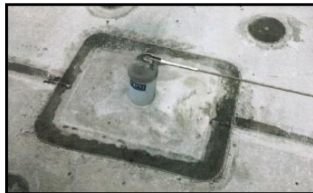
Roof-mounted Evolution End Post (New and Installed)
